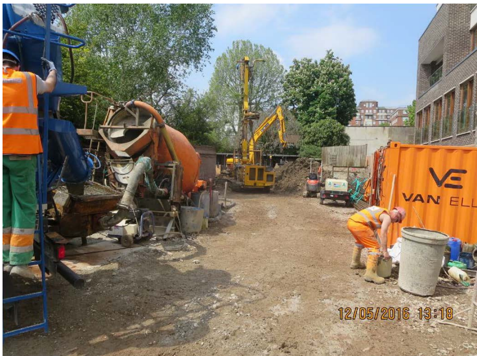
Previous building on site prior to demolition (top) and site as of May 2016 with previous building on site completely demolished (bottom).
